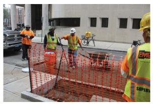
Workers from Emerge Connecticut Inc. construct a bioswale near the intersection of Wall and Church streets in New Haven in October.
