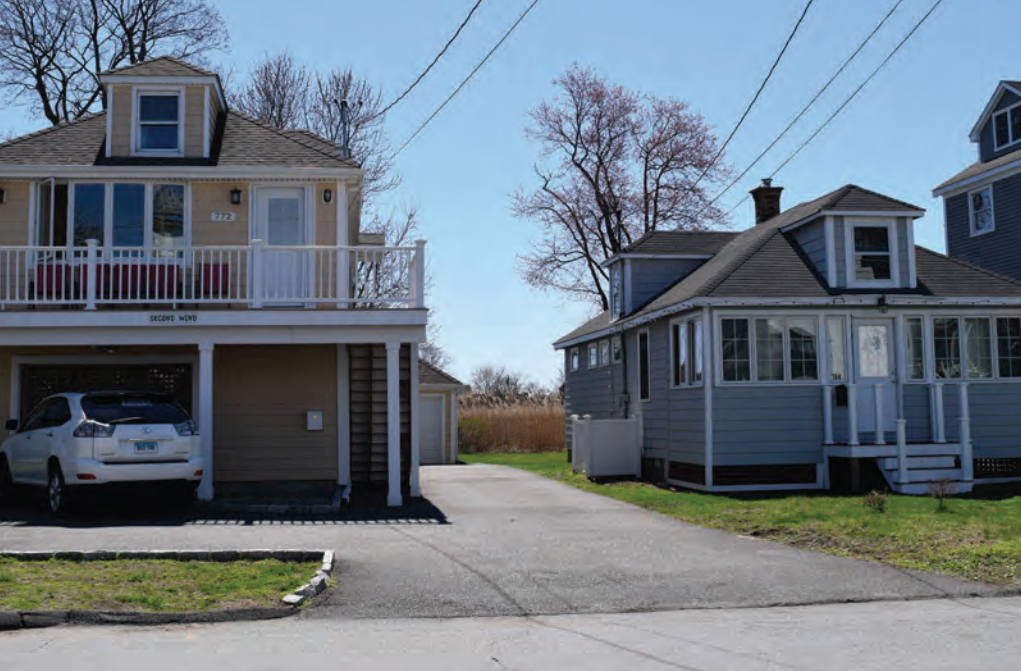
Two homes in Fairfield illustrate the contrast between those elevated after Superstorm Sandy, like the one at the left, and those that were not, like the one at the right. Photo: Nancy Balcom.
